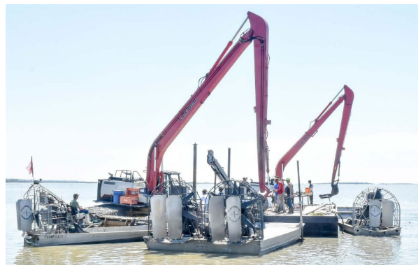
Figure 2 – Debris Field Excavation (Photo: NTSB)
